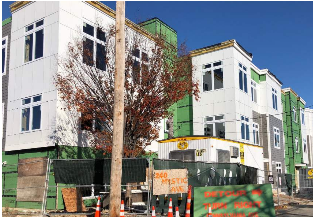
60 Cross Street East (Construction Photo)
